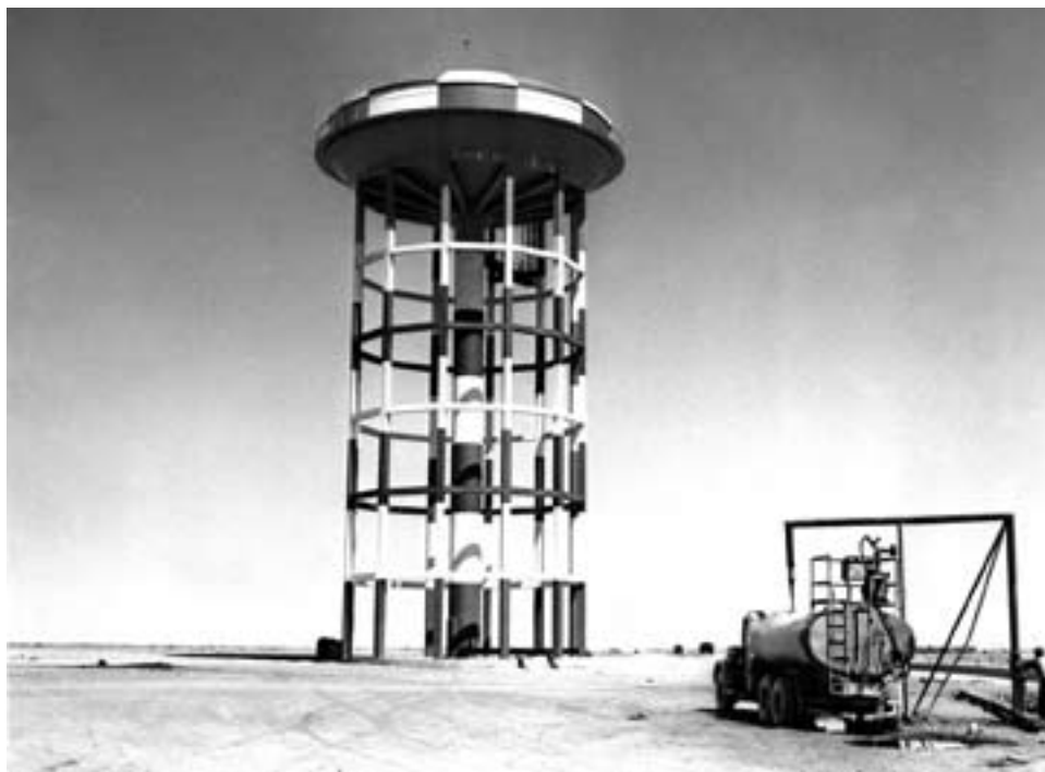
Elevated water tower at the Benguérir air base
