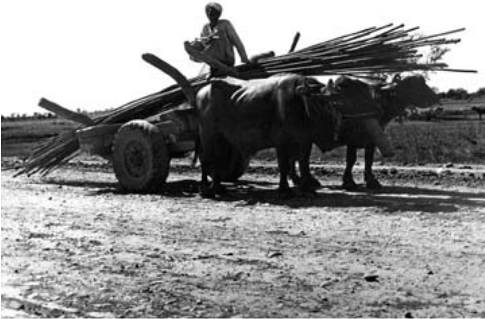
Local workers using animals to carry materials to construction sites at the Kharian cantonment
