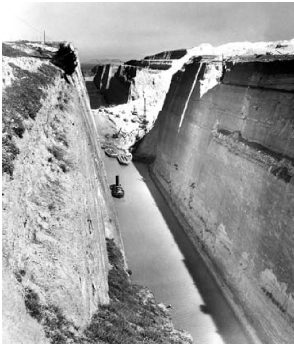
By April 1948, excavation of the Corinth Canal was over half complete.
