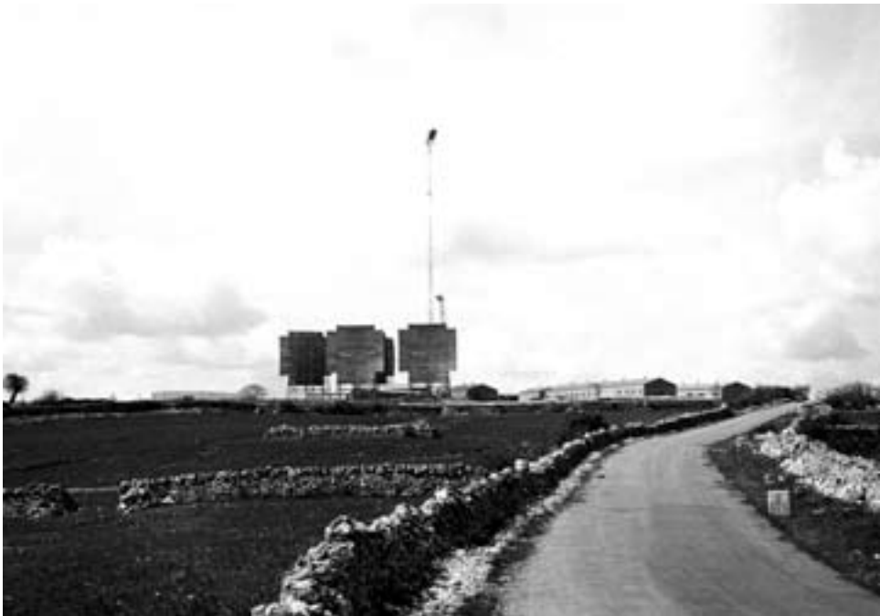
Troposcatter Site 20-A, Brindisi, Italy, 26 March 1965
