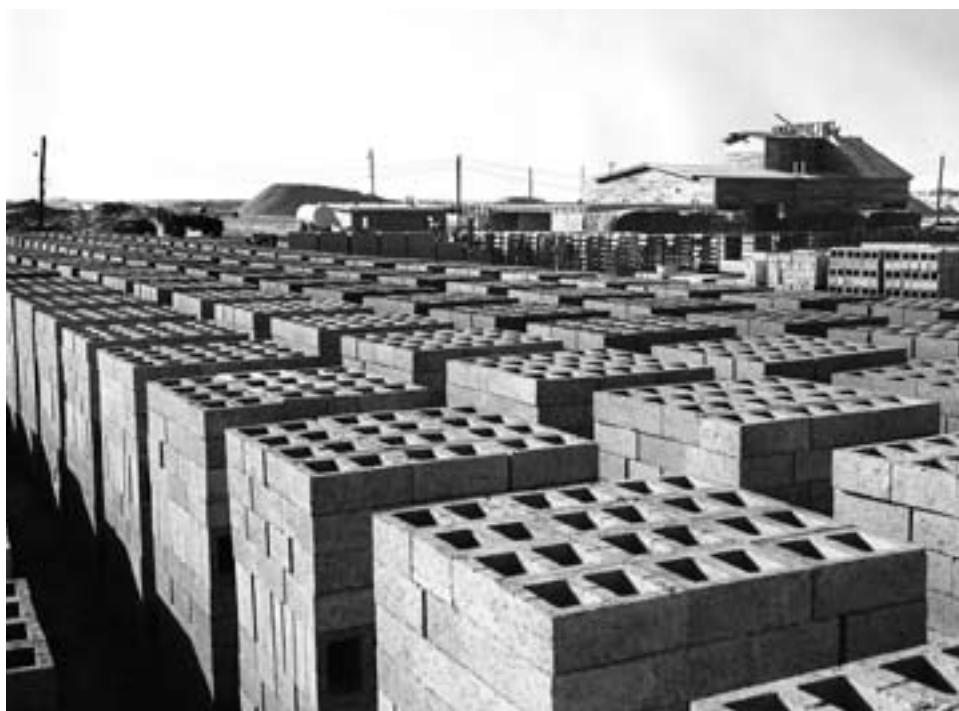
Concrete blocks drying in front of the batch plant at the Dhahran airfield
