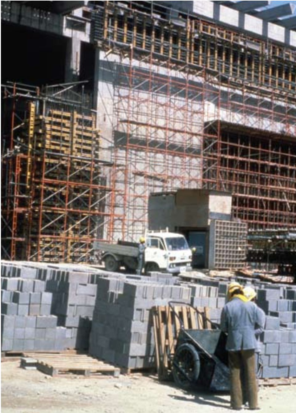
Main entry to the library/administration building under construction at King Abdulaziz Military Academy, early 1980s
