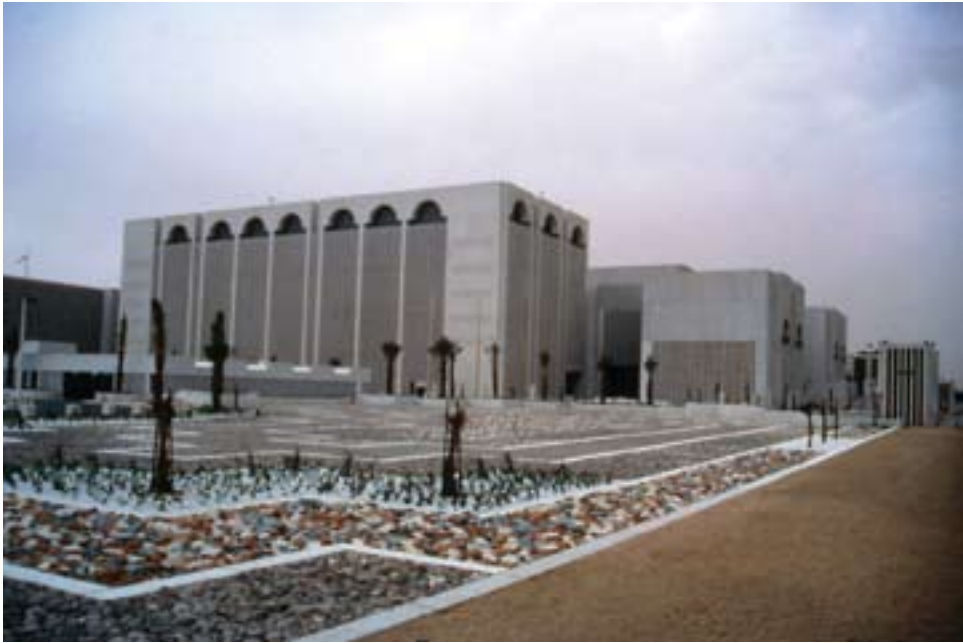
Headquarters, Ministry of Defense and Aviation, Riyadh, June 1986
