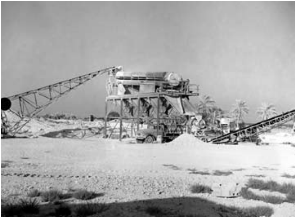
Rock-screening plant at Kharg Island
