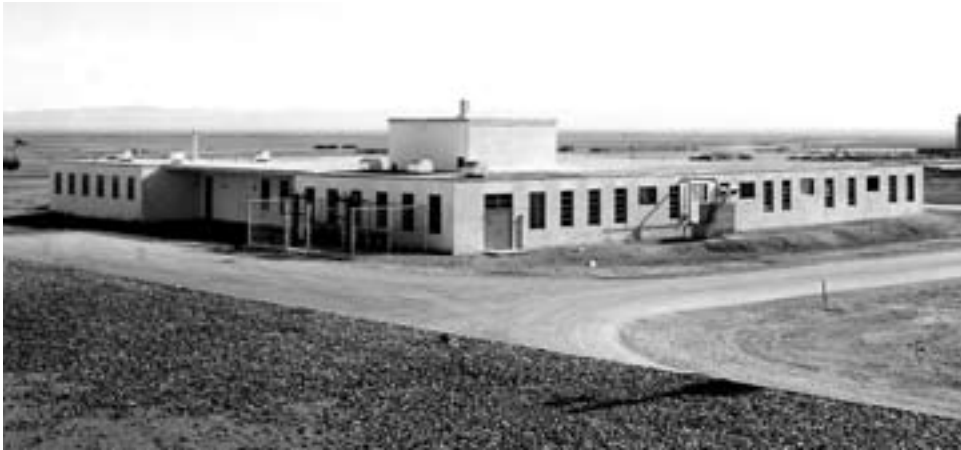
Armaments and electronics shop at the Benguérir air base, as seen from the parachute tower
