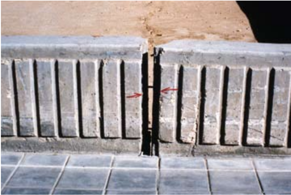
Settlement problems at King Abdulaziz Military Academy, shown here in 1990, led to some tension between the Corps of Engineers and Saudi officials.
