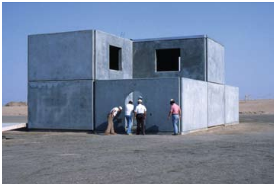
Test house built at Hafar al Batin using precast concrete panels, April 1979
