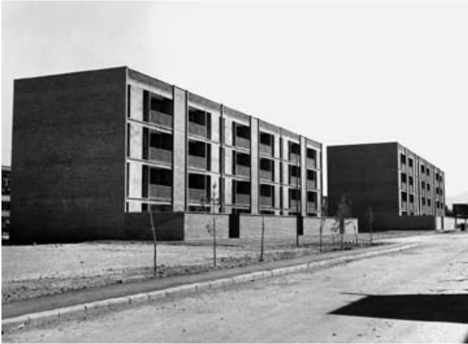
New apartment construction at Naziabad, ca. 1965
