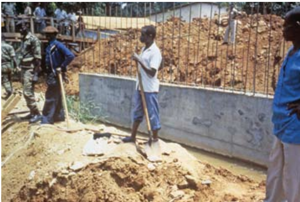
Construction workers at Camp du Kassai Bridge, Central African Republic
