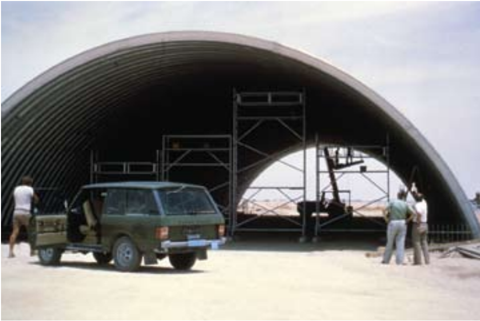
Aircraft shelter in Thamarit, January 1981
