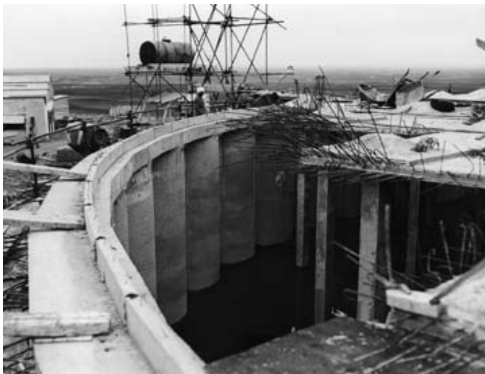
Water reservoir under construction at the Nouasser airfield, 16 December 1953
