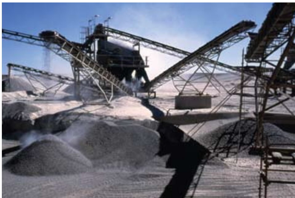
Rock crusher at Hafar al Batin, site of King Khalid Military City
