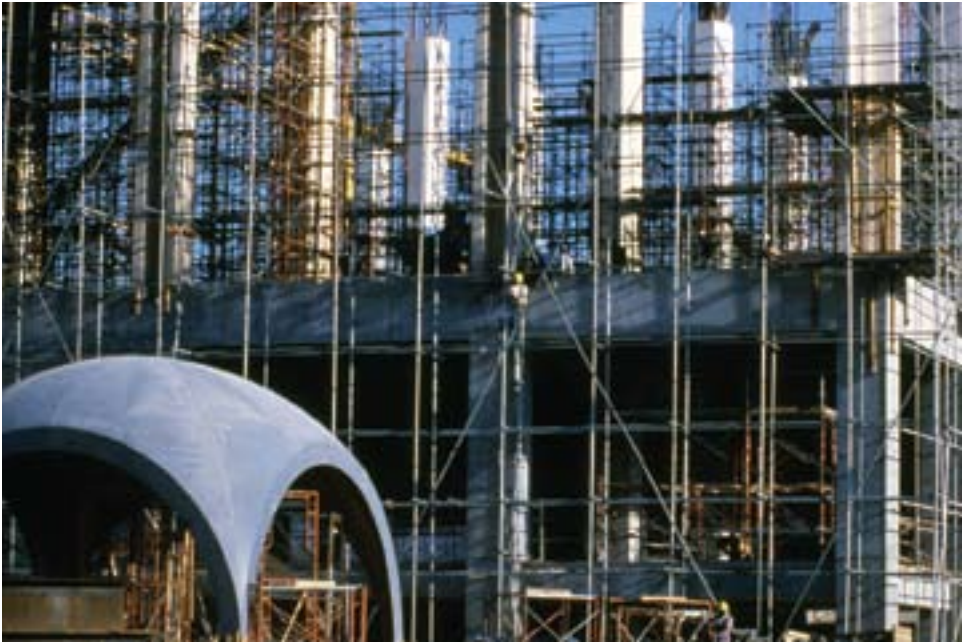
Centrum at King Khalid Military City under construction
