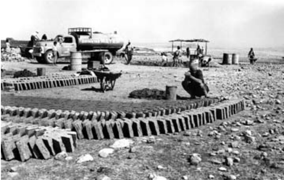
Bricks drying at the Dezful depot
