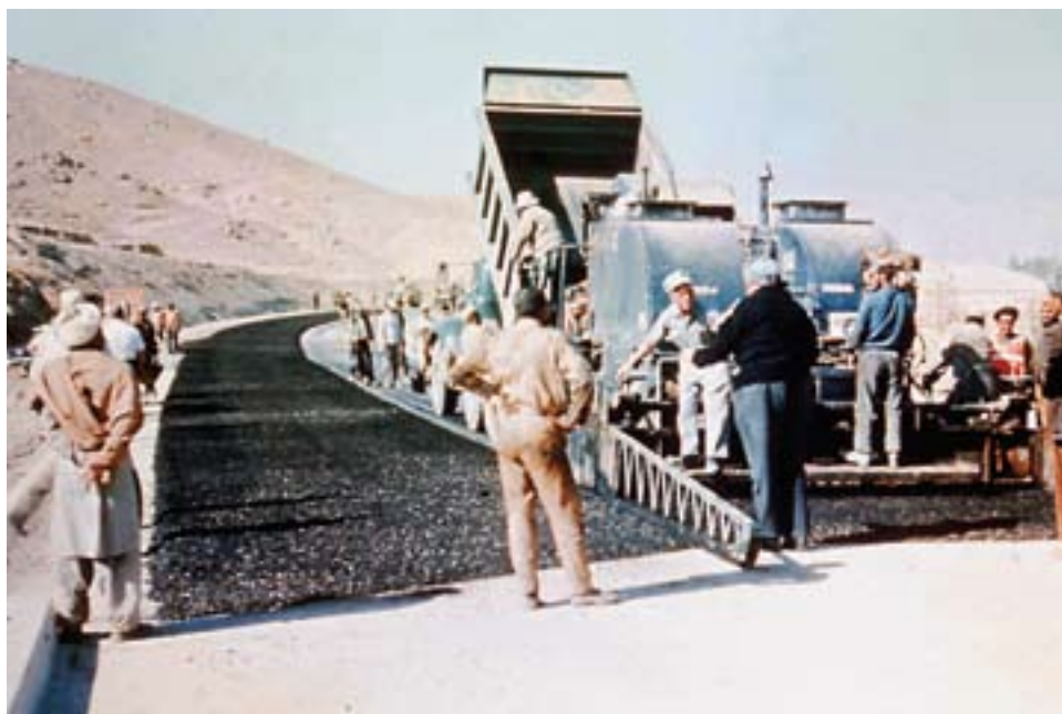
Laying asphalt during construction of the Afghan highway
