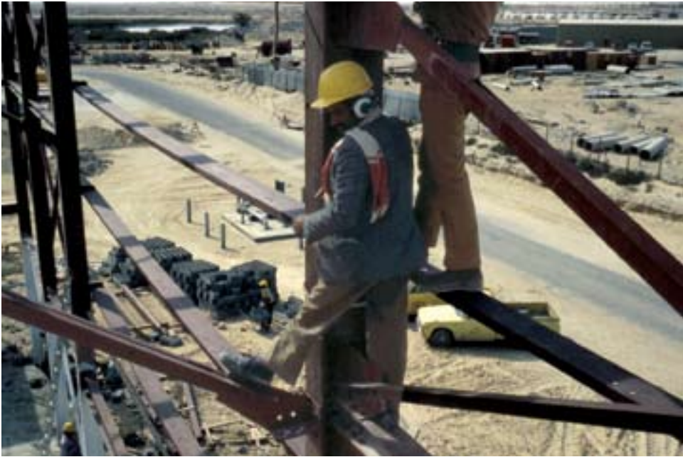
Construction for Peace Hawk, February 1978
