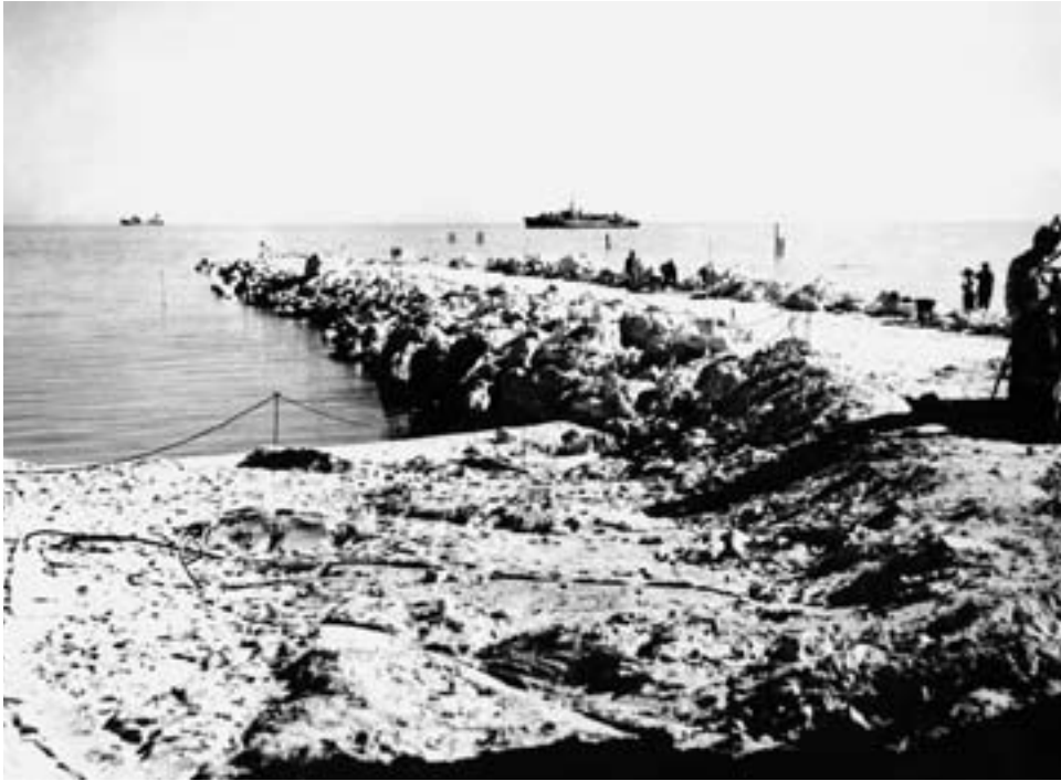
Breakwater on Kharg Island under construction, January 1962
