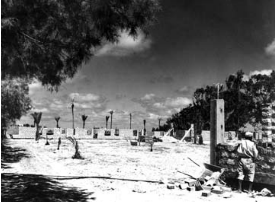
Contractors used native limestone in the construction of family housing at Wheelus Air Base, September 1951.
