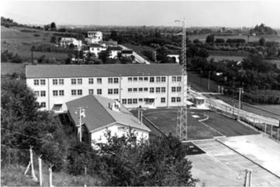
Mess hall ( front ) and barracks constructed in Vicenza
