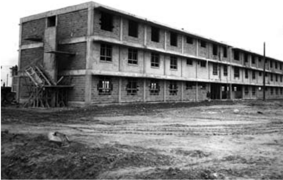
Airmen's dormitory under construction at Cigli Air Base, December 1961
