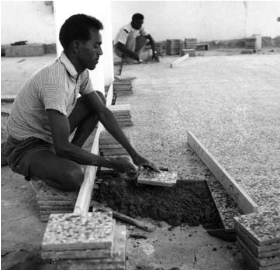
Workmen laying floor tiles in barracks at Asmara
