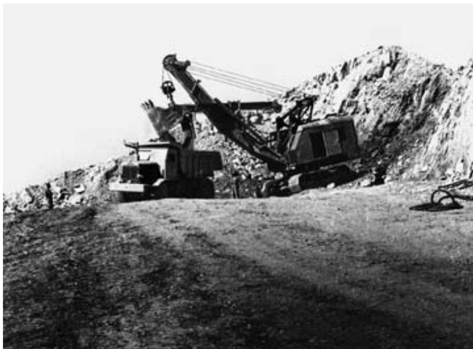
Construction of the Afghan highway, ca. 1966
