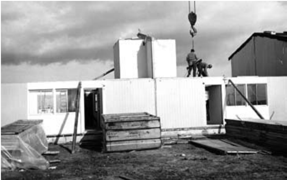
USAHOME apartment construction in Brindisi, March 1965
