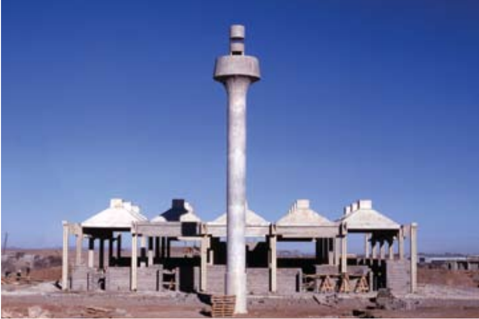
Mosque under construction at the Khamis Mushayt cantonment, December 1969
