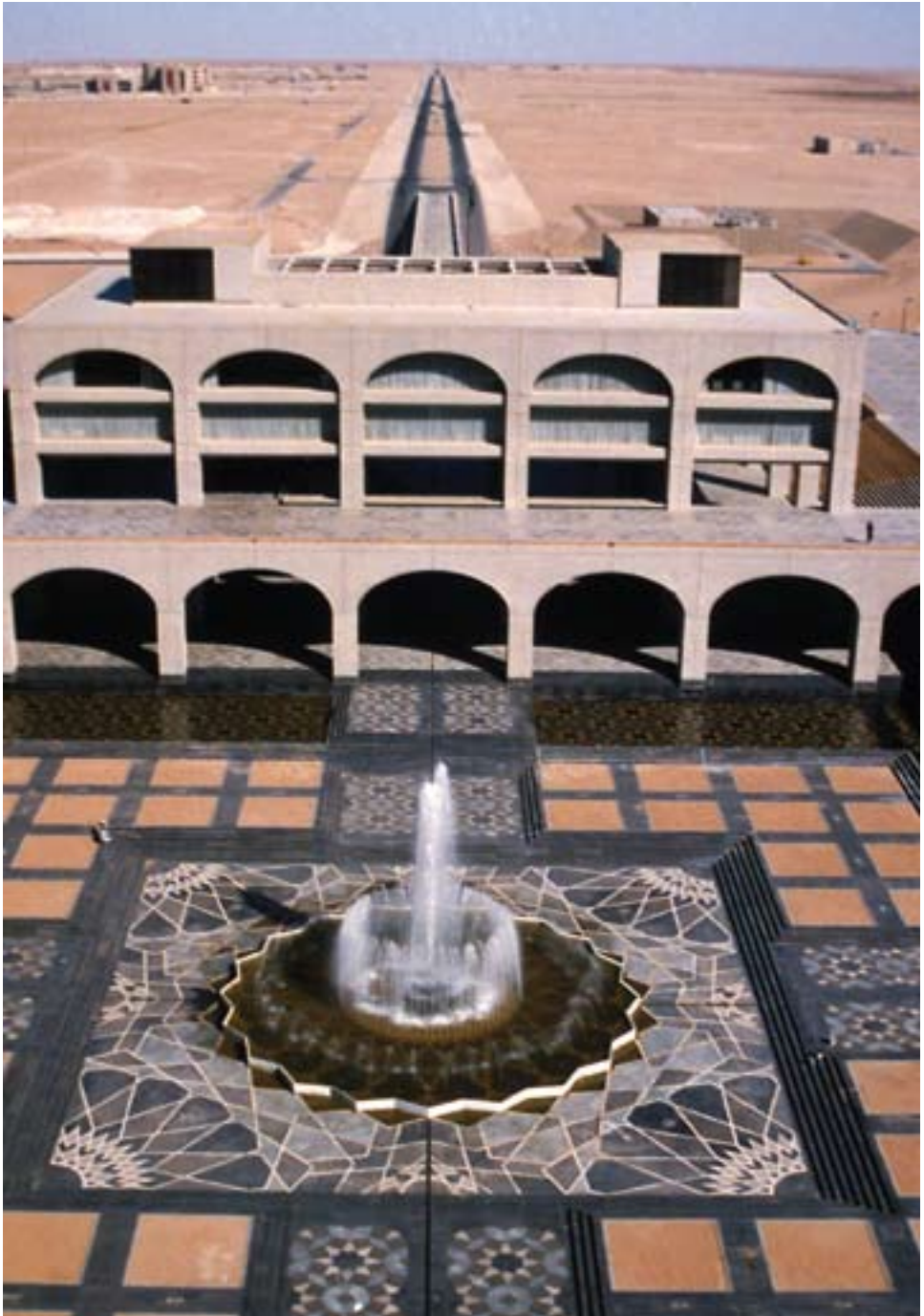
Completed centrum at King Khalid Military City, mid-1980s
