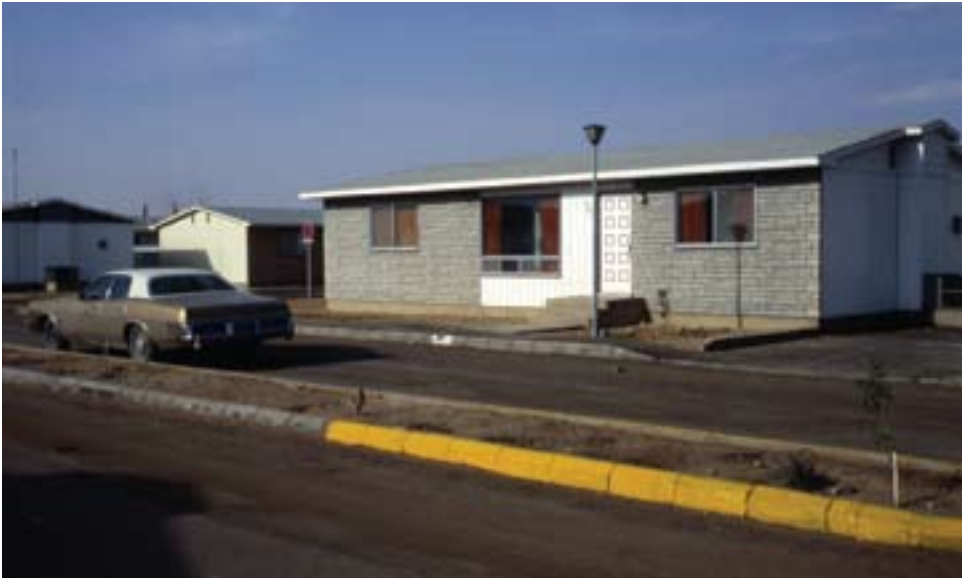
Housing built in Riyadh for lieutenants, ca. 1979
