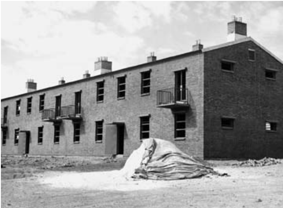
Noncommissioned officers quarters under construction at Quchan, October 1963
