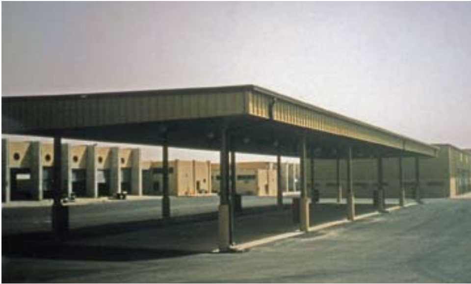
Sunshades at a Saudi Arabian National Guard facility, late 1970s
