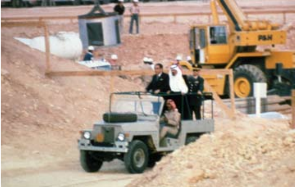
Prince Abdullah touring the construction site of the Saudi Arabian National Guard headquarters complex, 1977
